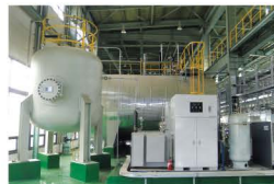
Pressure Maintaining System: Paju Combined Heat & Power Plant Construction Project Project Owner : Korea District Heating Corporation Contractor : Daewoo Engineering & Construction Pressure Maintaining System: 90m 3 x 2 units
