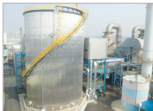
Pressure Maintaining System: Paju Combined Heat & Power Plant Construction Project Project Owner : Korea District Heating Corporation Contractor : Daewoo Engineering & Construction Pressure Maintaining System: 90m 3 x 2 units
