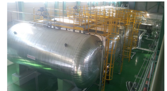
Construction of Korea Midland Power Co., Ltd.
