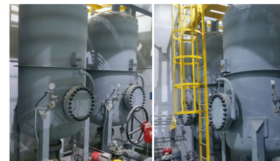
PanGyo Combined Heat & Power Plant Expansion Project
