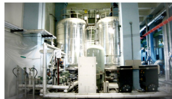
Southeast District Distribution Complex CES Construction Project
