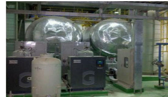
Goyang Samsung Combined Heat & Power Plant Construction Project
