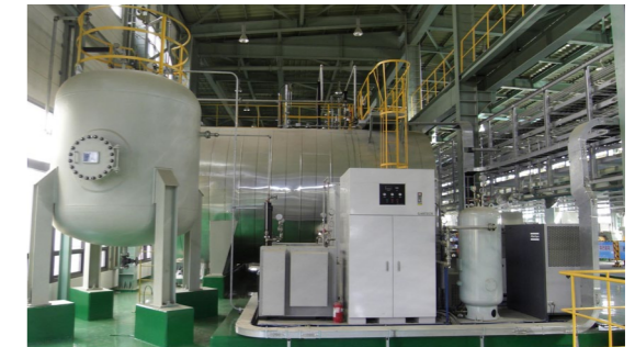
Paju Combined Heat & Power Plant Construction Project
