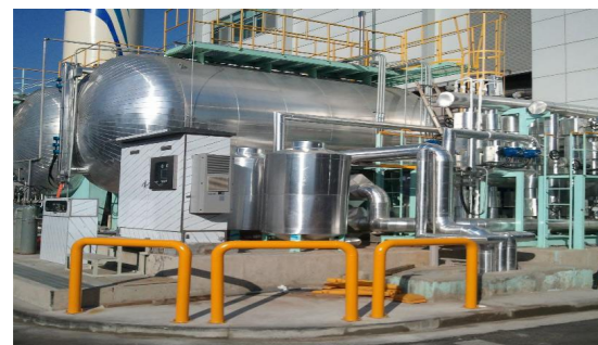
Osan Combined Heat & Power Plant Expansion Project
