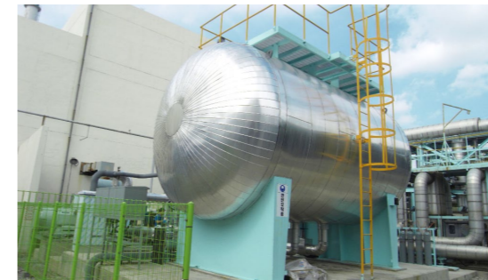
Osan Combined Heat & Power Plant Expansion Project
